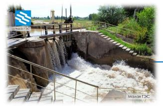
Location of SHPP selected with the greatest slope with maximum use of hydro potential of the river.
